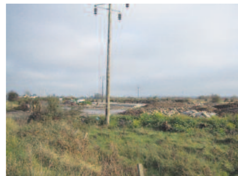
Eyesore created by tipping on the bog at Allenwood
