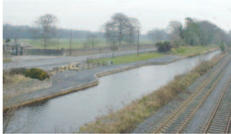
Views from Pike Bridge onto the Royal Canal
